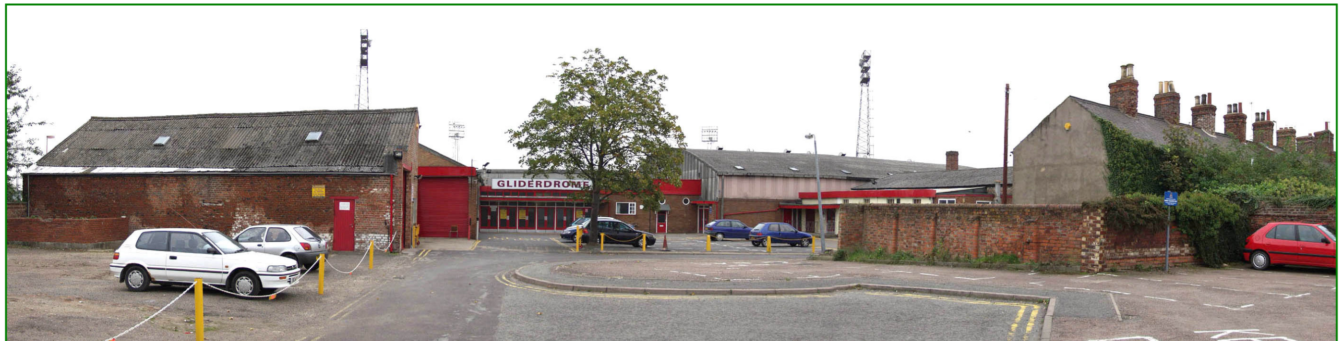
PLATE 4: View from footway on John Adams Way, looking east.
